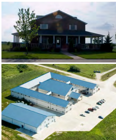
Enjoy your residential experience at either one of HCC's housing facilities: The Ozark House (top) for women or the Dorm for men.
